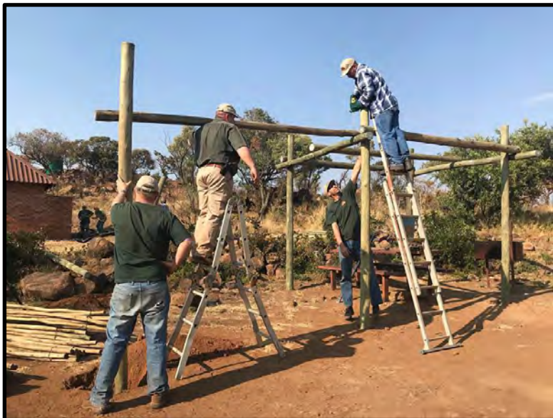
Construction of the second half and roof of the shade structure.
