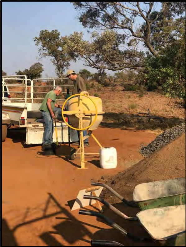
Pathway team, who loaded and poured load after load of concrete
