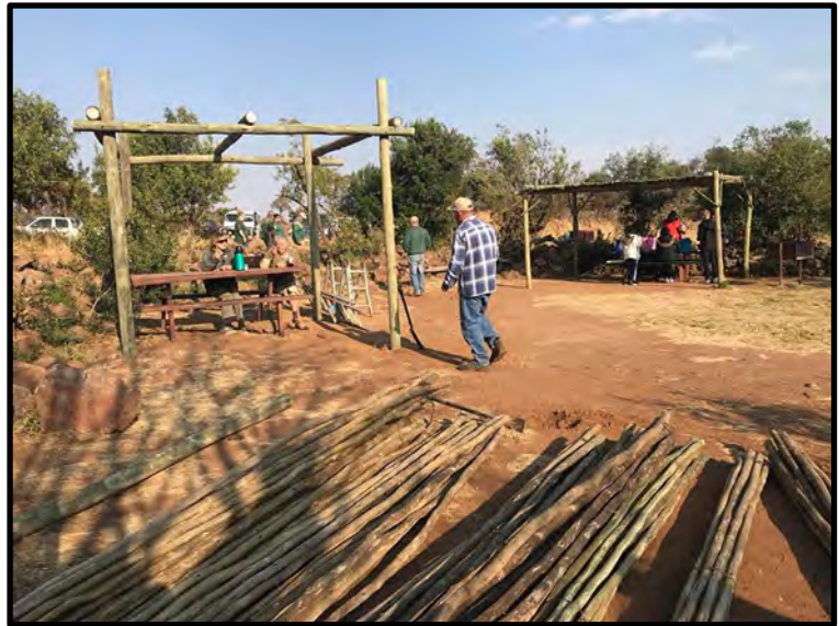
Construction of the second half and roof of the shade structure.
